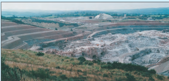
Open-pit at Kingscourt gypsum mine. Evidence of earlier underground workings can be seen in lower centre. (Courtesy: Gypsum Industries Plc).
